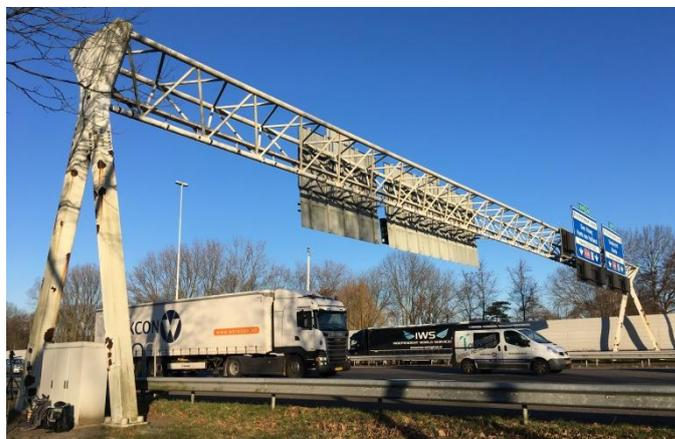
**Figure 1.1** A typical sign gantry in the Netherlands with signboards and electronic signs
