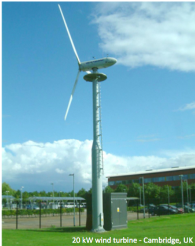
(a) 20 kW prototype brushless DFIM based wind turbine. Courtesy of [40].
