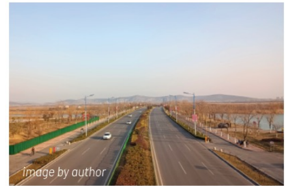
Connected to the city by highway G105.
