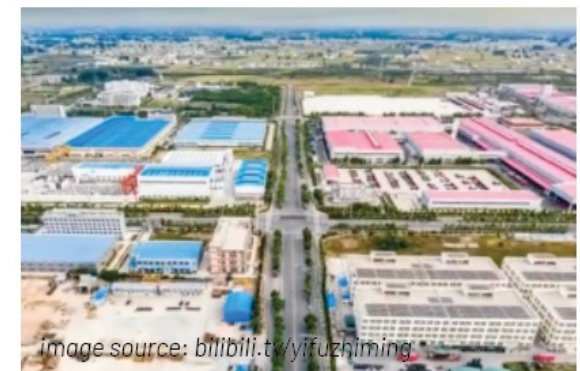
The construction of the industrial park sprawls into agricultural land.
