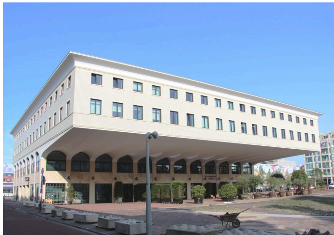
Figure 11: A building with a 16 meter overhanging canopy (Wind, 2024)
