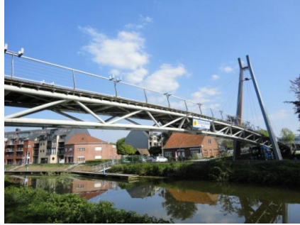
Figure 1 The footbridge in Ninove, Belgium.
