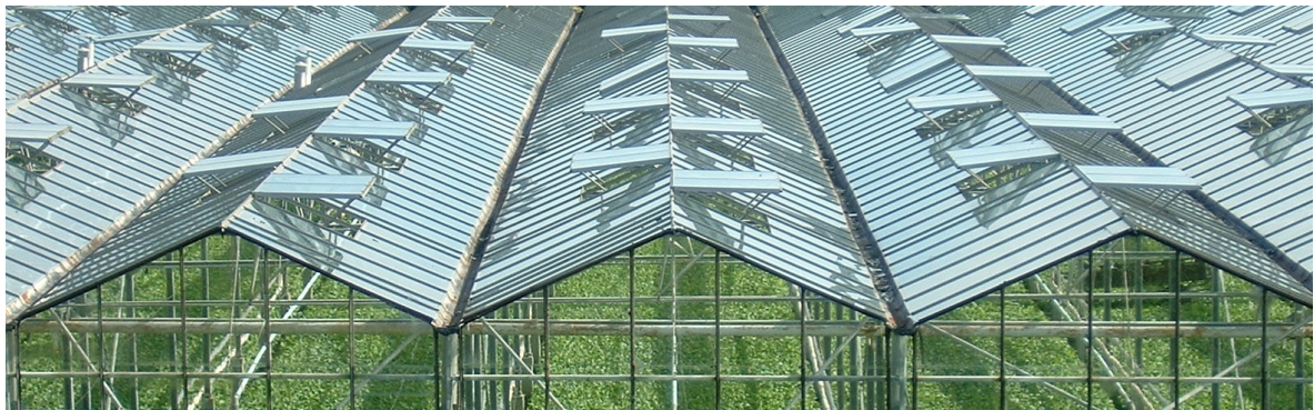
Figure 2-1: Typical multi-span Venlo type greenhouse [19].
