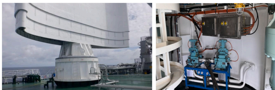
Fig. 26. Leakage diagnosis and analysis of the sail hydraulic system [156].
