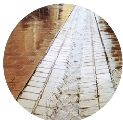
Gutter brickstones
