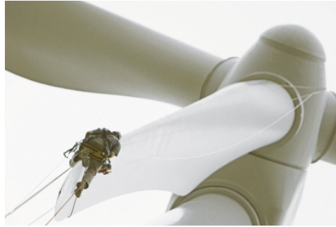
Figure 2.3: Rotor blade maintenance: Rope access
