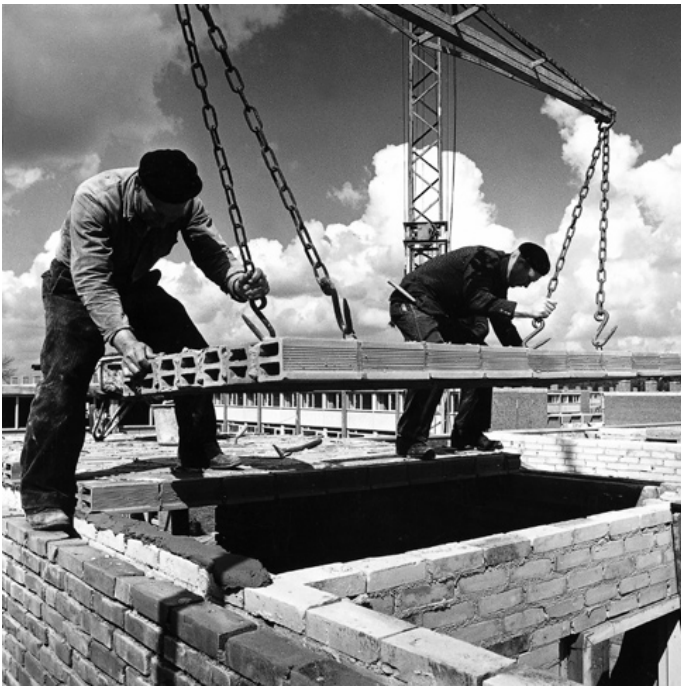
workers assembling prefabricated brick slabs with the help of a building crane (source: Wouter van Heusden, gemeentearchief Emmen)
