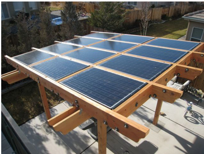
Pergola with built-in PV panels (Dickson, 2012)
