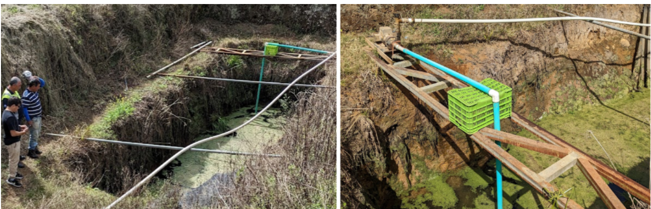
Figure 26: Informal well with a depth of around 7 meters used only by the lettuce farmer. Notice the abundance of algae, a sign of eutrophication
