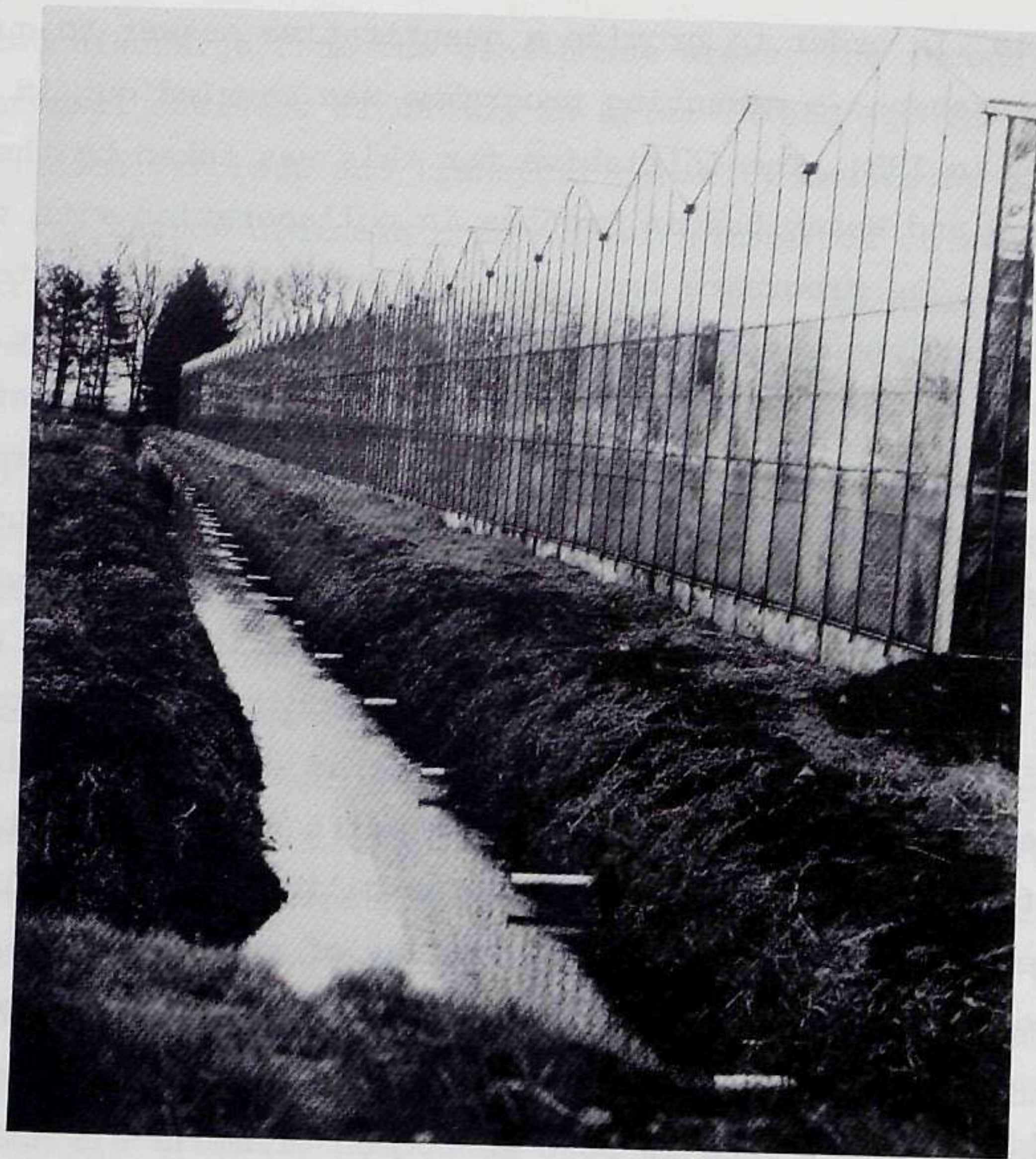
The drainage situation in Erica Ig
