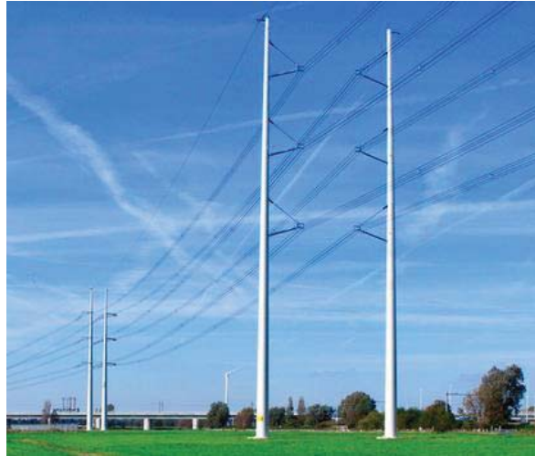
Figure 1-1: Windtrack power pylon
