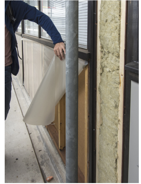
Fig. 83. Refurbishment of facade panels
