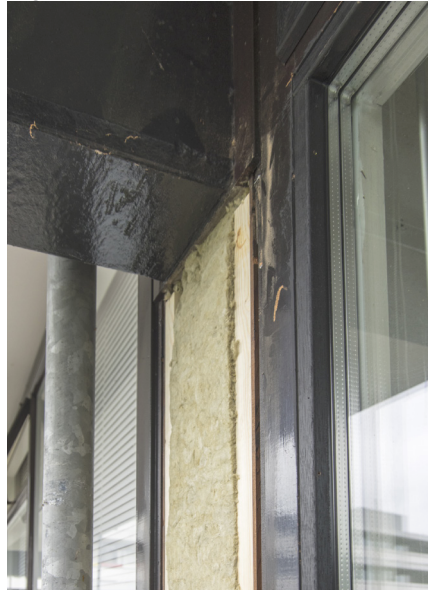
Fig. 82. Insulation of concrete structure
