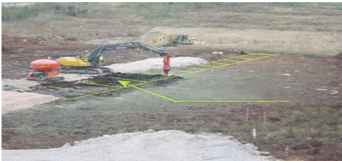
Figure 2.5; The division of the area in blocks prior to stabilisation (Allu Finland Oy, 2007).
