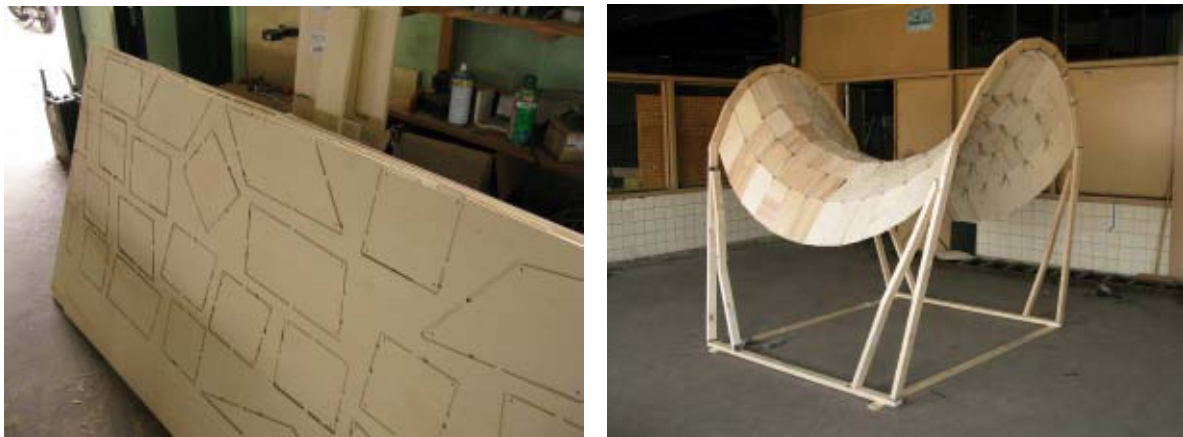
Figure 4: Panels and Work in Progress
