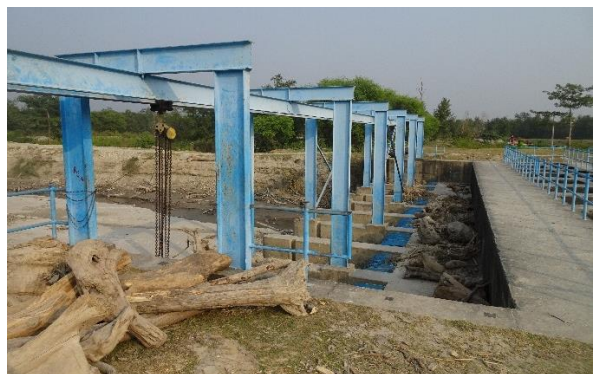
Irrigation intake blocked by debris
