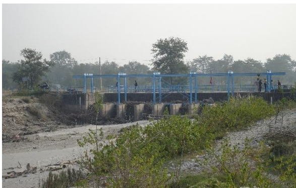
Irrigation intake blocked by debris, looking downstream
