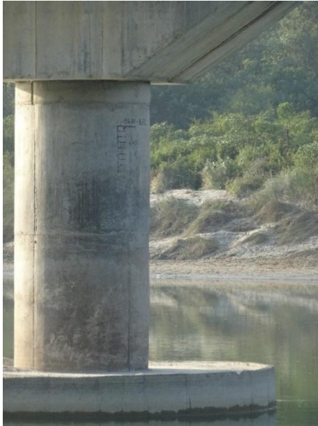
High flow level marked on bridge support
