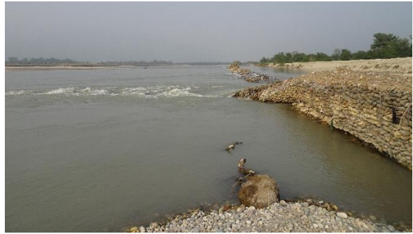
Dam breach at irrigation intake, looking upstream
