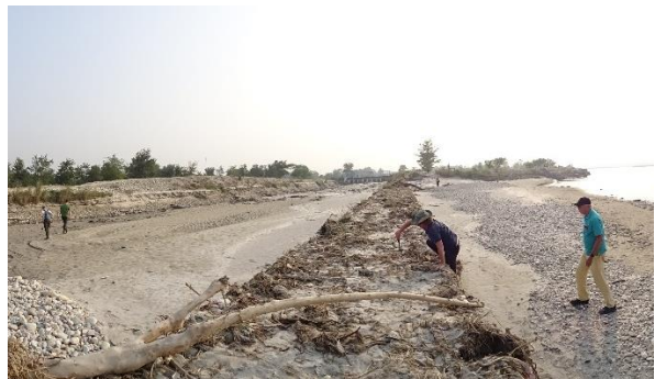
Sediment deposition behind dam breach, (downstream)
