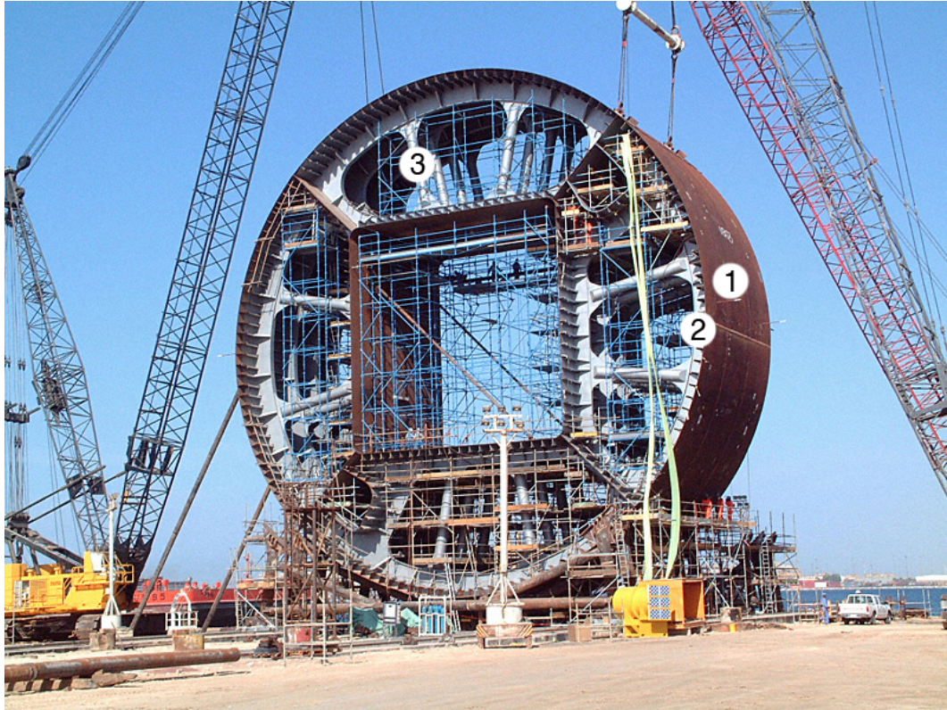
Figure 3.2: Platform ring with numbered components used to construct table 3.2 [4]
