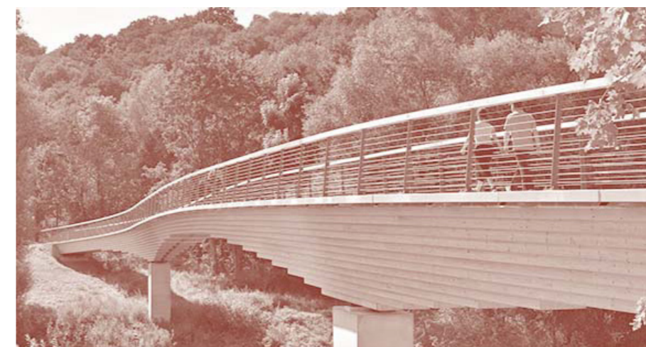
A: Overhang 30° Protection 240mm extended Concrete deck above Glulam, 30° to vertical rain protection (DIN 68800)
