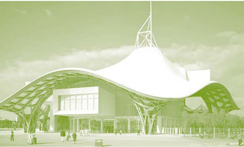
D: Water Resistivity Double beam Larchwood as column due to its water resistivity
