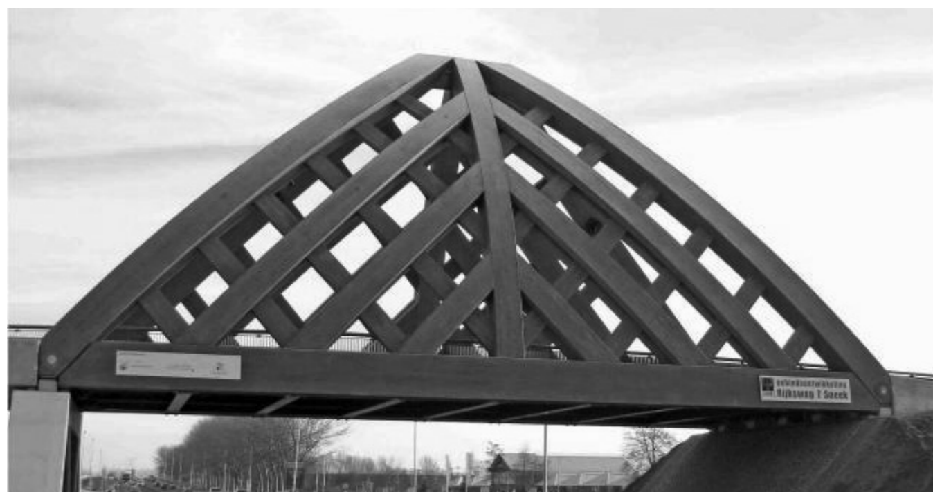
Fig 2.6: Sneek bridge, spanning 40m across the A7, with cycling and traffic lanes is capable of withstanding 65 tons of load.
