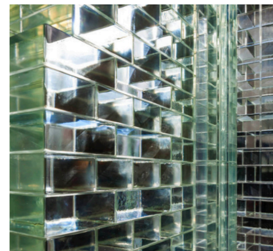
Figure 41. Adhesive connections in cast glass: Crystal Houses/MVRDV. From "ArchDaily," by Scagliola, D. & Brakkee, S., 2016 ( https://www.archdaily.com/785923/crystal-houses-mvrdv ).
