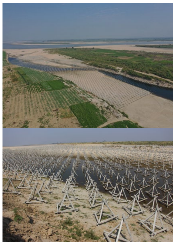
Figure 3 Channel suppression using porcupines in Ayeyarwady River, Myanmar
