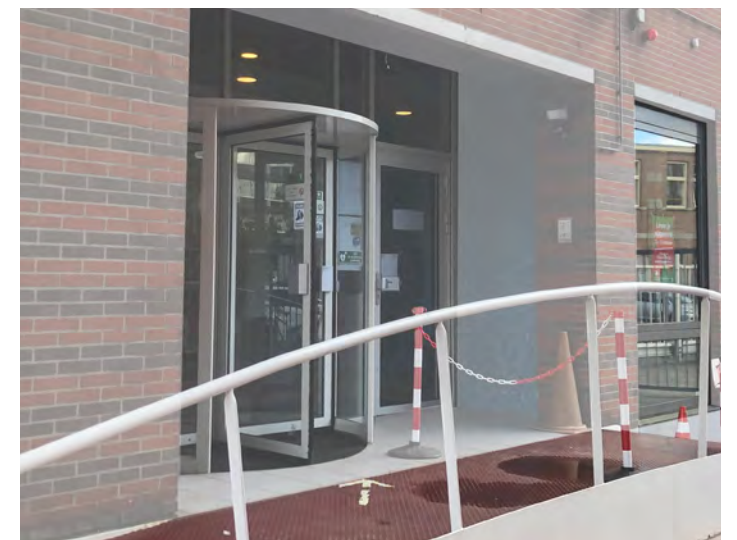
Fig. 89b: Steel ramp and aluminium door
