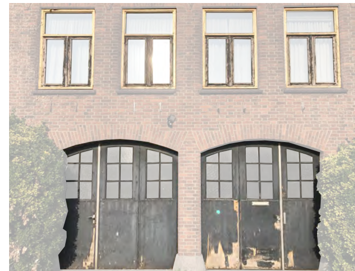
Fig. 101a: Wooden window and door frames 1940 build.
