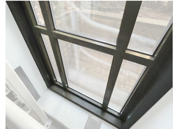
Fig. 100b: Aluminium window frame 1933 building
