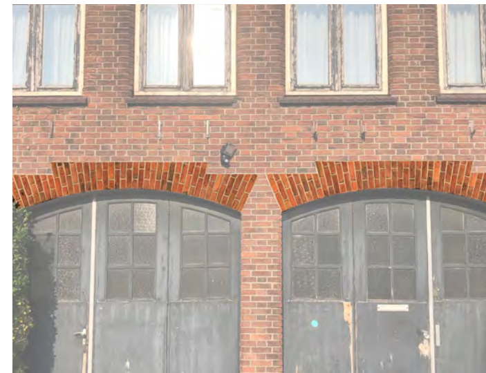
Fig. 71a: Segmented arches 1940 building
