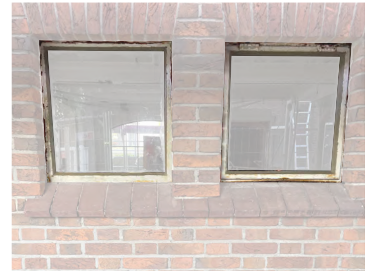
Fig. 101b: Steel window frames 1940 building
