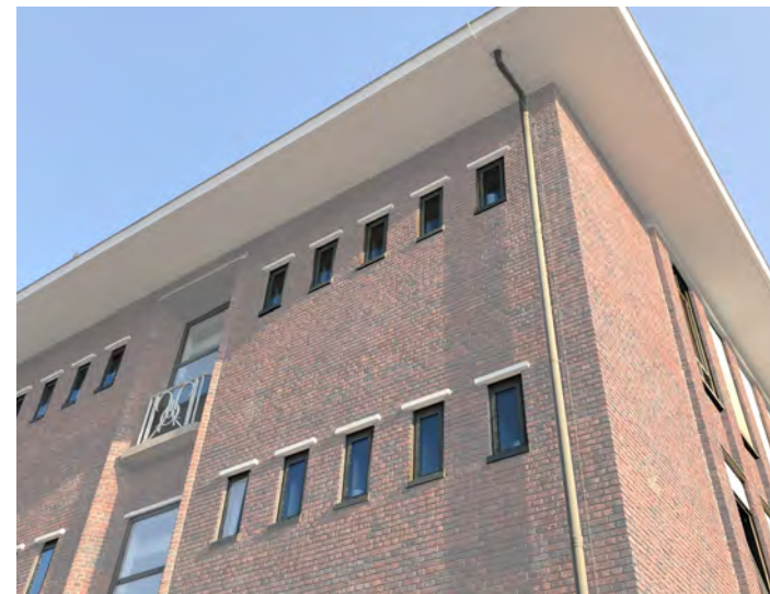
Fig. 88a: Steel windows and fence 1933 building
