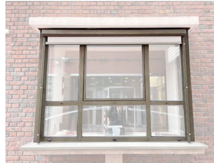
Fig. 100a: Aluminium window frame 1933 building
