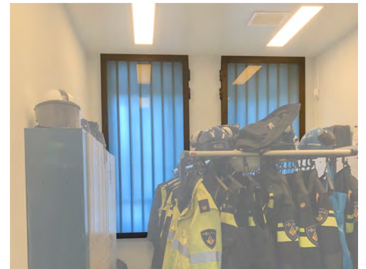
Fig. 88b: Steel window frame and cell fences
