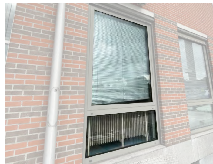
Fig. 123a: Tilt and turn + fixed window 1994 building
