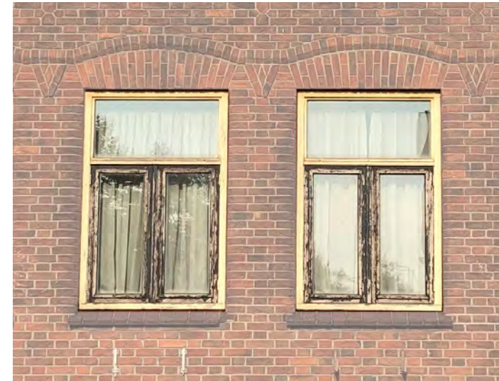
Fig. 90a: Wooden window frames 1940 building
