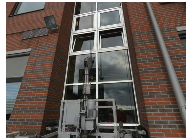
Fig. 102b: Steel window frames 1994 building
