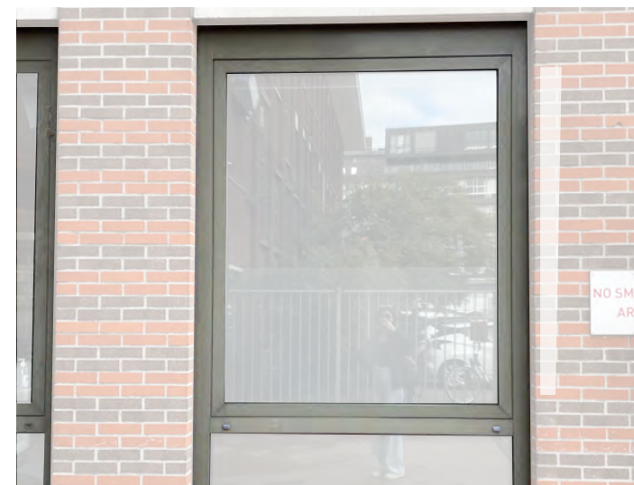
Fig. 102a: Aluminium window frame 1994 building
