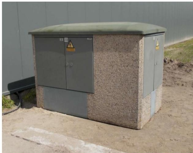
Figure 5-1: Example of a compact secondary substation
