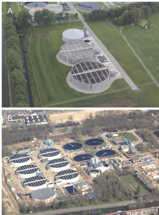
Figure 11.1 Nereda® wastewater treatment plants in the Netherlands in (A) Garmerwolde (140,000 P.E.) and (B) Utrecht (430,000 P.E.). In Utrecht the new 6-tank Nereda® facility (in operation since 2019) is visible on the left with part of the old abandoned plant on the right.
