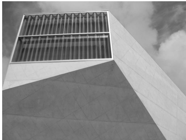
Figure 4: Corrugated facade in Casa da Musica (Nijssen 2008)
