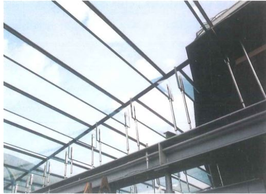
Figure 32: ING office, Budapest (Nijssse 2003)
