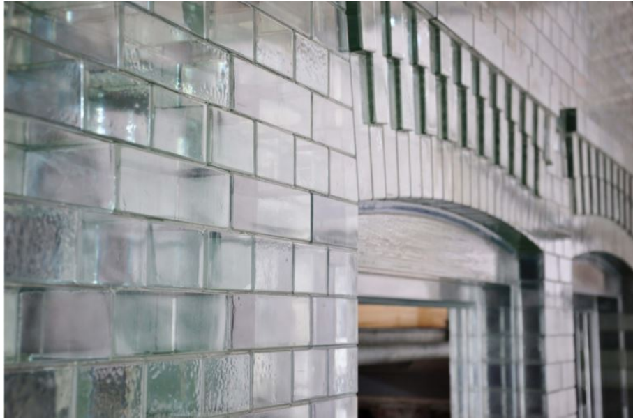
Figure 24: Close-up of the executed facade of the Crystal House in Amsterdam (Oikonomopoulou, T. Bristogianni, et al. 2016)
