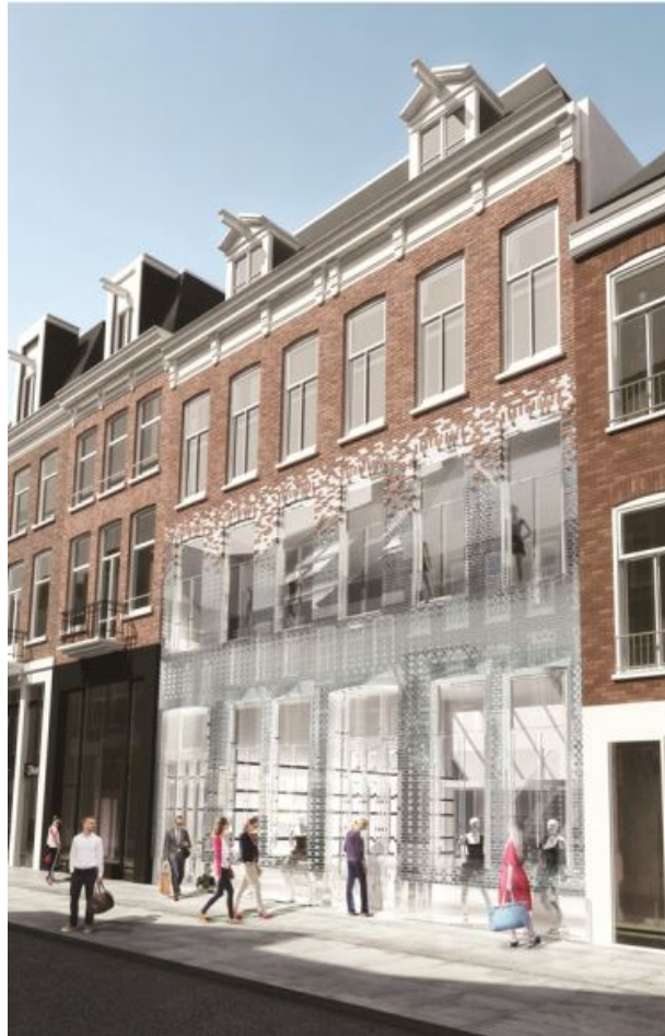
Figure 9: An impression of the Crystal House glass brick facade (Oikonomopoulou, T. Bristogianni, et al. 2016)
