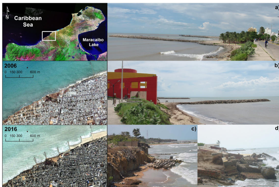
Figure A.1: Riohacha Guajira study case. a-b) groins building along city promenade. c-d) erosion related damages after groin construction (oblique photos, Satellite and Terraserver images for 2006-2016 period) (Rangel-Buitrago, N., et al., 2017)
