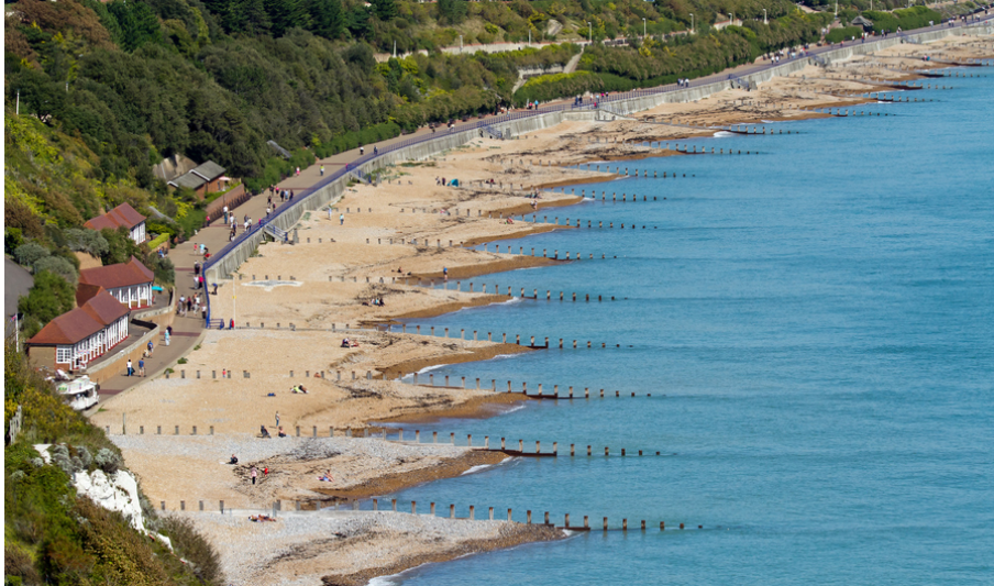
Figure 5.12: Wooden groynes in Eastbourne
