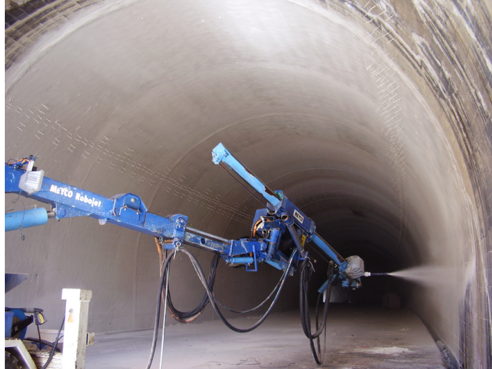
Figure AH.24: Epoxy spray equipment [92]
