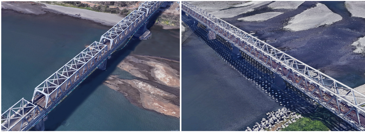
(a) Tohoku Shinkansen Tonekawa Bridge [4]
