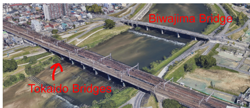
Figure 1.3: Bridges near Biwajima [4]
