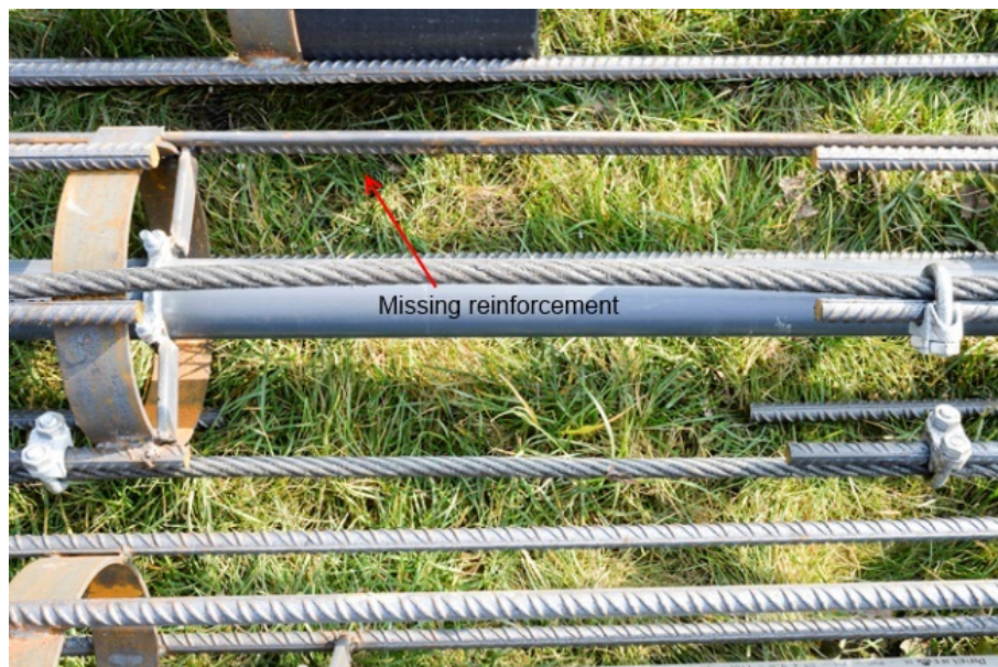
FIGURE C.3: Procedure for installing a crack. Picture provided by Deltares.
