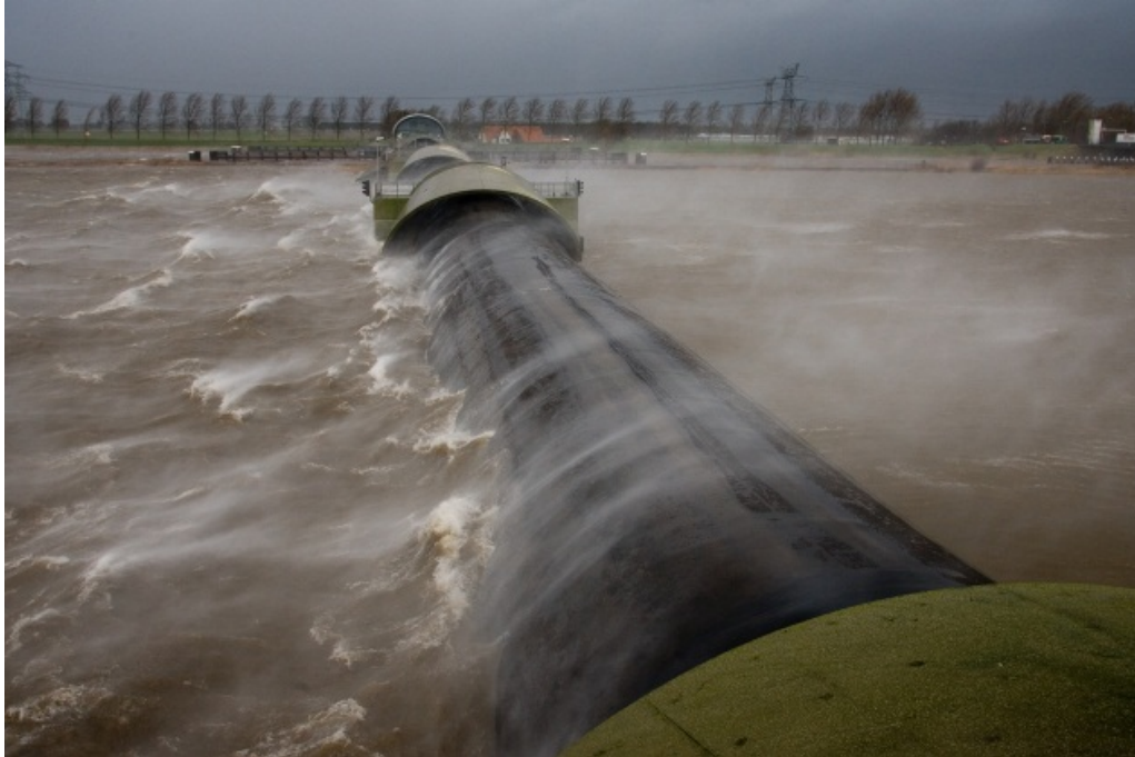
Figure 4: The inflatable rubber barrier at Ramspol [5]
