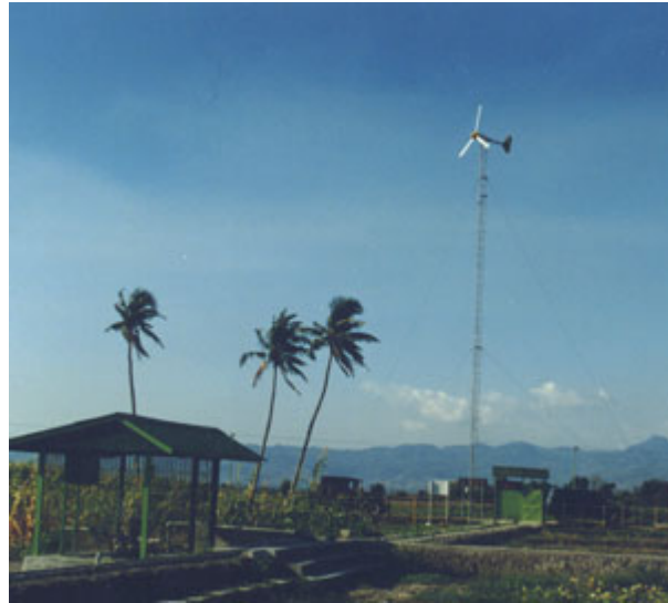
(b) Electric wind pumping [38]
