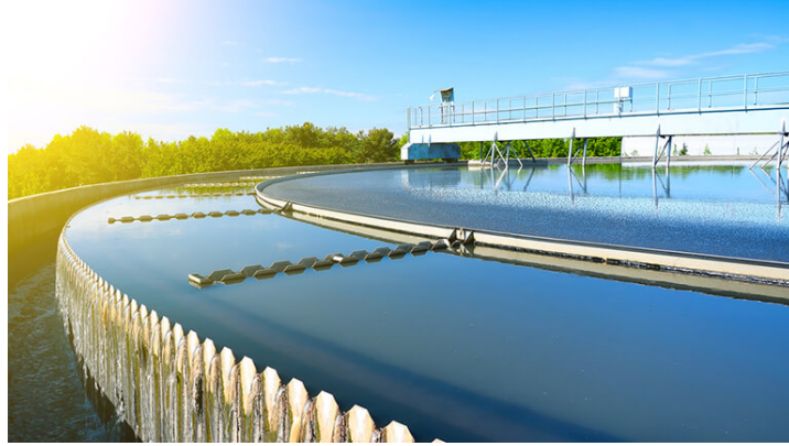
Figure 5.1: Water-treatment plant overview. Source: Rovatti [109].
