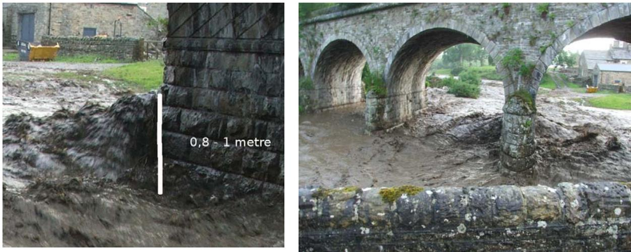
*Figure 4-2: Example of a super-elevation in front of bridge piers located in a river bend and showing a lateral velocity gradient : 0.8 to 1 metre in front of the left bank pile, about 0.5 in front of the central pile and neglectable on the right bank pile. July 2007, Mill Burn, Northumberland, Great-Britain.*
