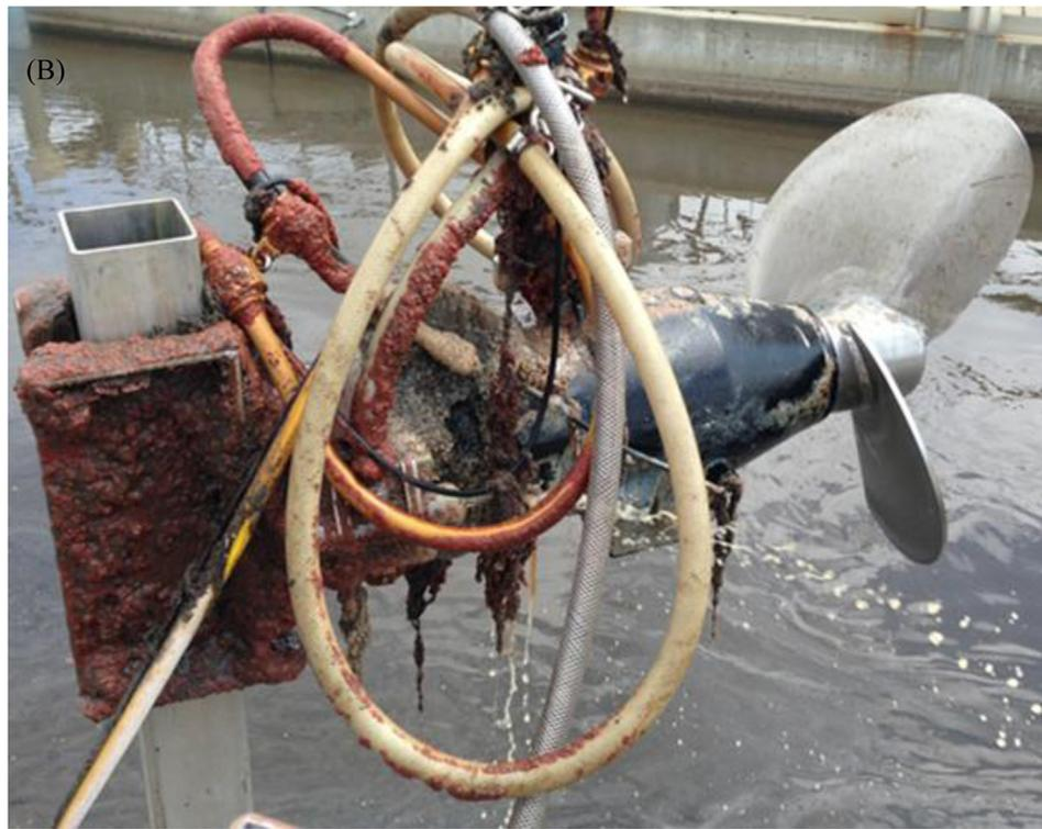
Fig. 1. (A) Schematic diagram of the full-scale nitritation-denitritation process treating separate centrate with glycerol addition. (B) Red biofilm on the surface of anoxic mixer.
