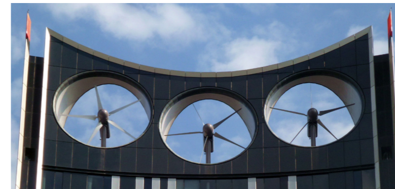
Figure 158: Wind turbines in building design -1 Note. Reprinted from De Groene Energie Maatschappij (n.d.).
