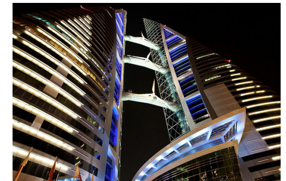
Figure 158: Wind turbines in building design -2 Note. Reprinted from De Groene Energie Maatschappij (n.d.).
