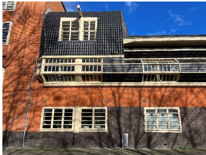
Figure 3.11: The façade on the Zaanstraat opens up to the street with big windows cantilevering over the sidewalk.
