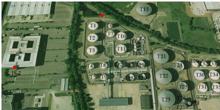
Figure 4.5 Layout of the Buncefield oil depot before 2005, the UK (Chen et al., 2020a)
