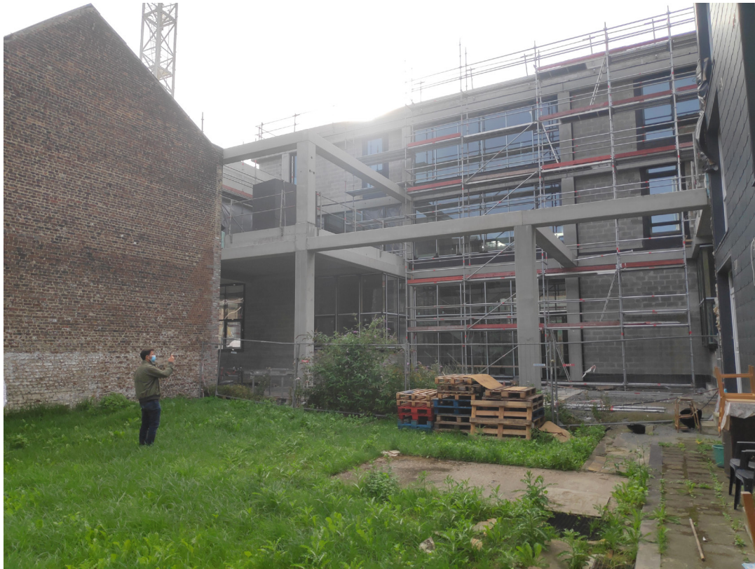
Photograph of the current condition of the social court. A blind facade of the old atelier building facing the facade of building b. The space has no purpose, no signs of occupation, only nature is taking over.
