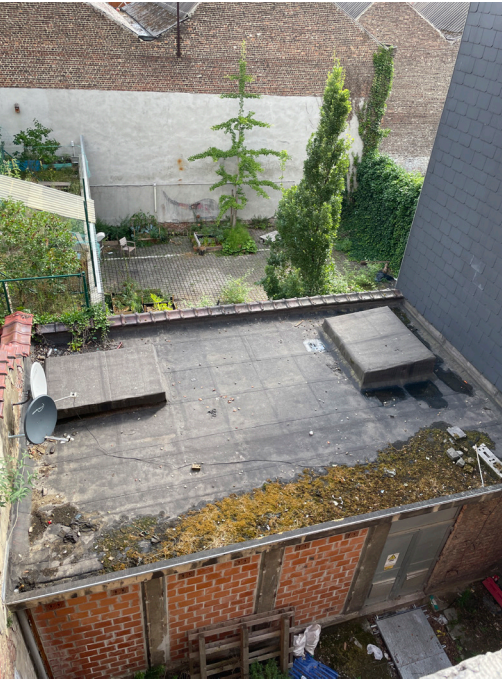
Shed from top view, in the background parking area of the daycare centre. (Image from Pierre Renard - Kaderstudio)
