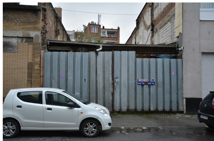
Interior tucked away and covered by metal plates
