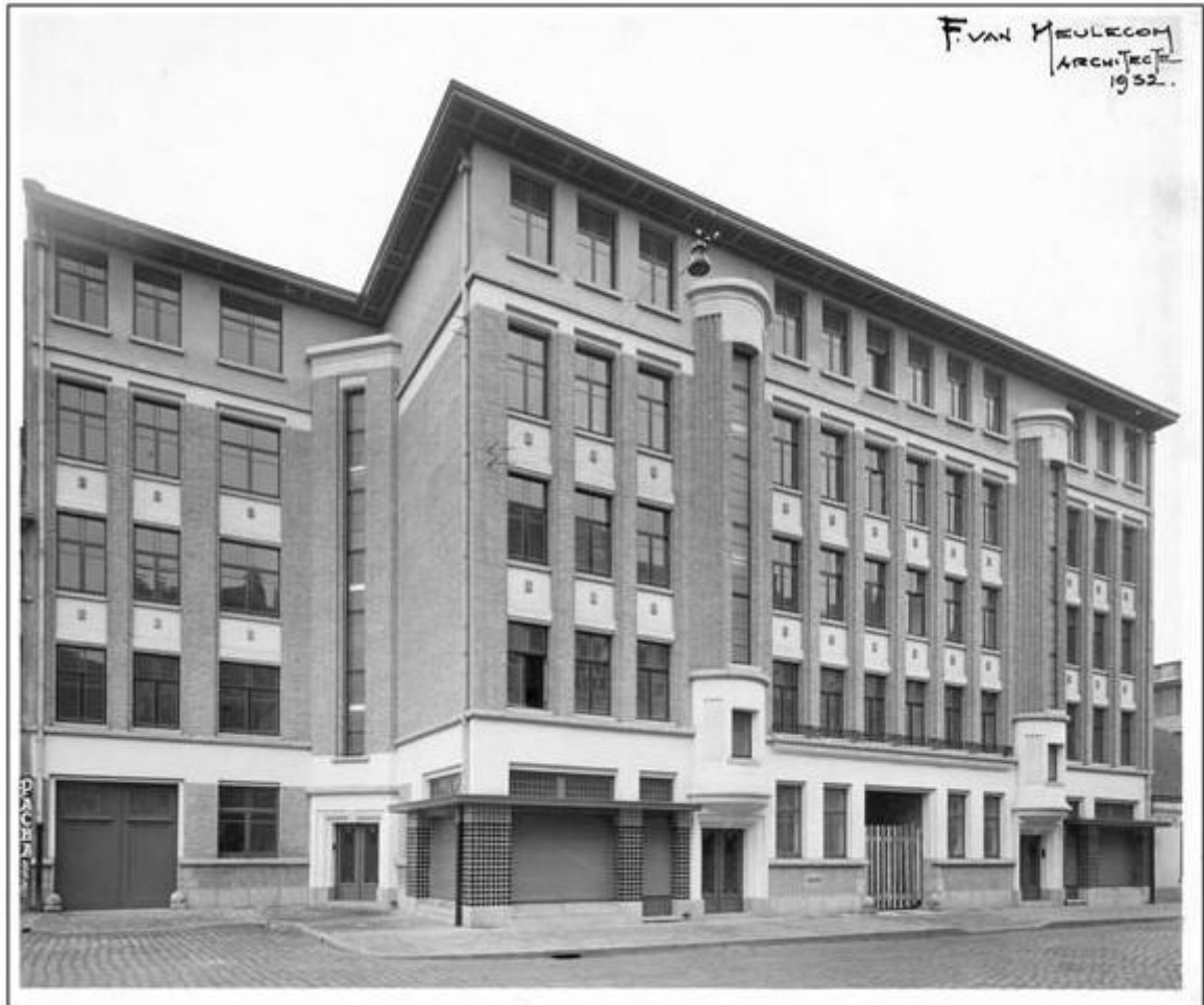
Rue de Liverpool 14-22 facade upon completion. The image shows the beauty and richness of the building in its prime age. Ornament, brickwork and lot of openings define this facade.
