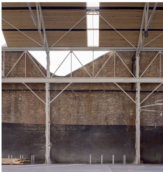
Shed accessibility from the De Grote Hal side.
