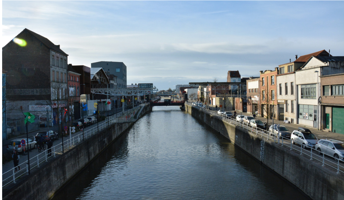
View from the bridge to the canal and the site. Calm yet busy atmosphere.
