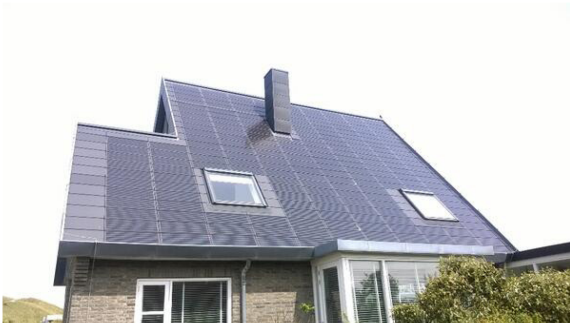
Figure 28. Integrated PV panels on a house in the Dutch town of Callantsoog (Van der Leun, 2016).
