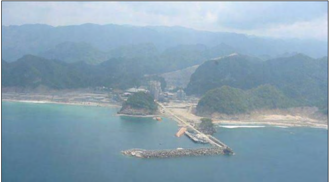
Figure 2-15 Helicopter view of breakwater Lhok'Nga, source [47]
