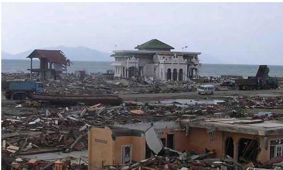
Figure 3-10 Banda Aceh port area. Mosque in Ulee Lheue, directly on the coastline. Close to this location the 12m inundation depth was measured. Almost all (simple) buildings were destroyed [67].
