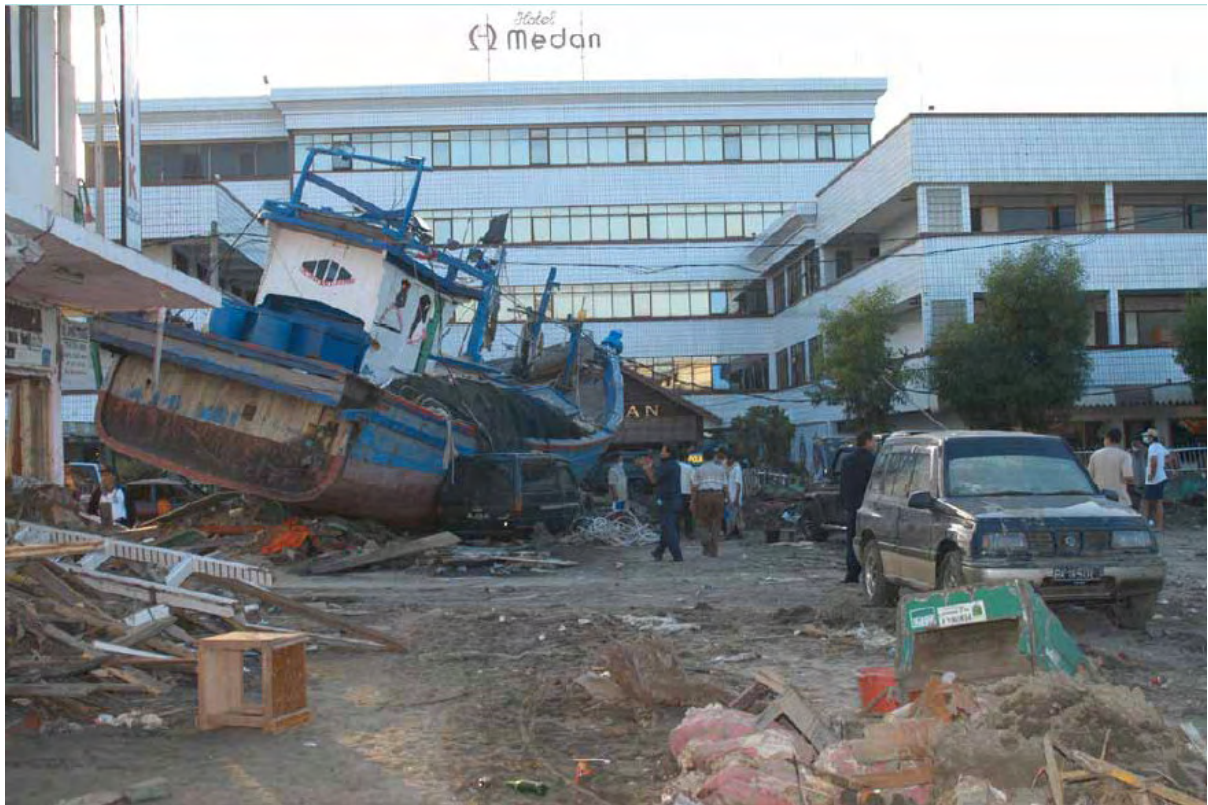
Figure 3-11 Banda Aceh. Downtown, approx. 3km inland, close to the Great Mosque. The boat was most probably moored in the river next to this site. A lot of debris is in the streets but the (concrete) buildings do not show structural damage [67].
