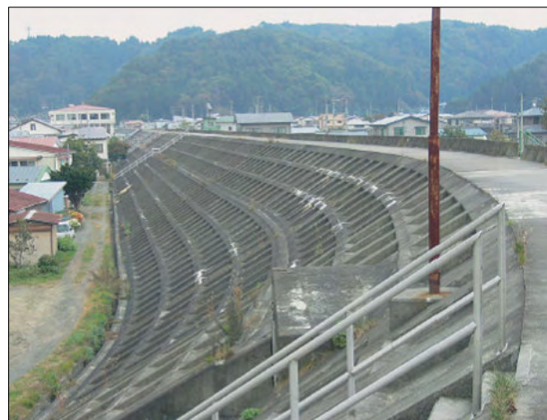
Figure 2-12 Seawall of 10m height in Taro, Japan [10]
