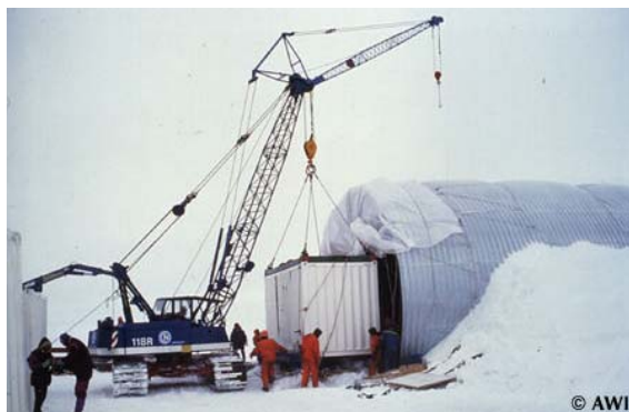
FIGURE 43: construction of NM 1991/1992 ( photograph: AWI )
