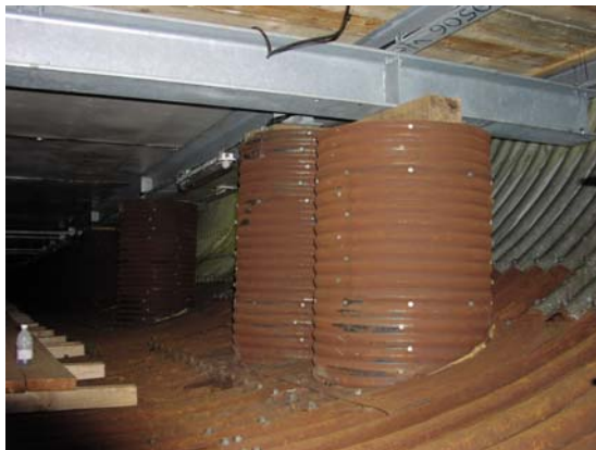
FIGURE 37: platform structure at Neumayer Station (photograph: M. Takata)
