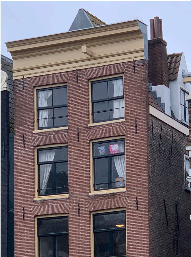
Zoom-in wooden cornice top of facade. Own picture
