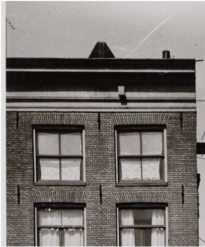
Roof structure in 1936. Source: Stadsarchief Amsterdam, 1936.
