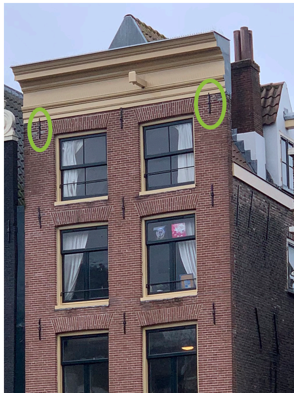
Wall anchors. Own picture.
