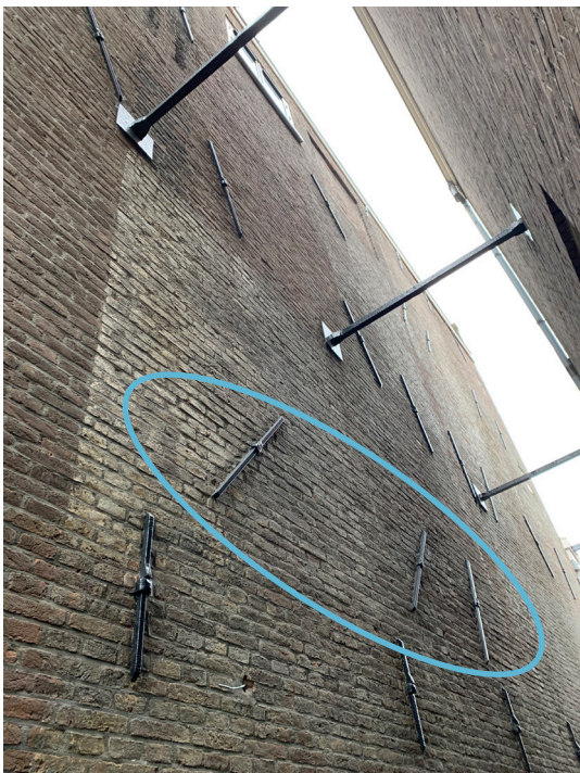
Wall anchors North facade. Own picture.
