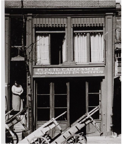
Lower East facade in 1936. Source: Stadsarchief Amsterdam, 1936.
