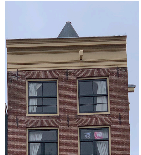
Roof structure in 2021. Own picture.
