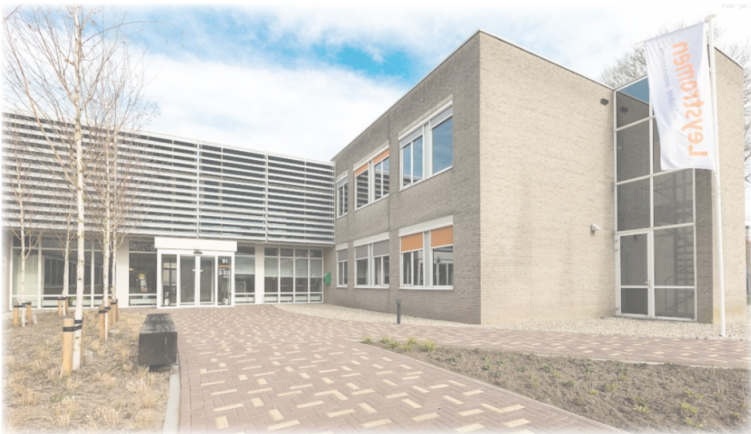
Case 4 Office building Rijen
