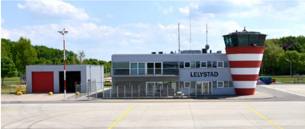
Figure 5.2: Left fire brigade, right terminal building with ATC tower [Schiphol group, 2014]
