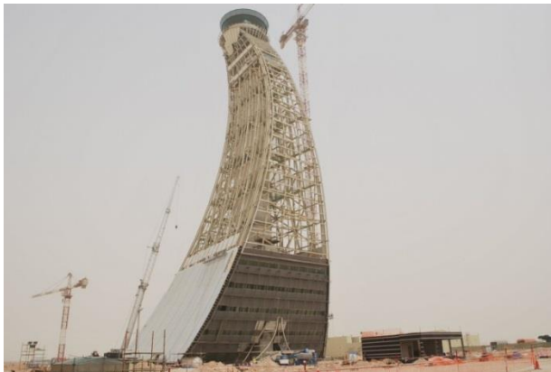
Figure 3.11 Abu Dhabi tower under construction. [panoramio, 2011]
