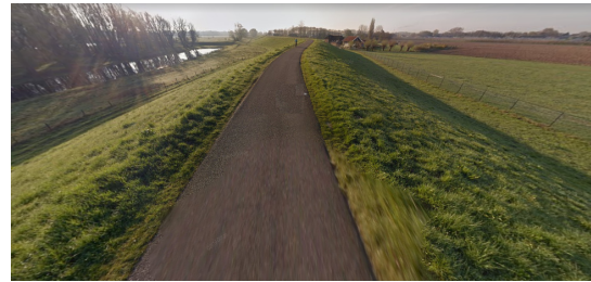
(b) Impression of the landside slope of the Waaldijk
