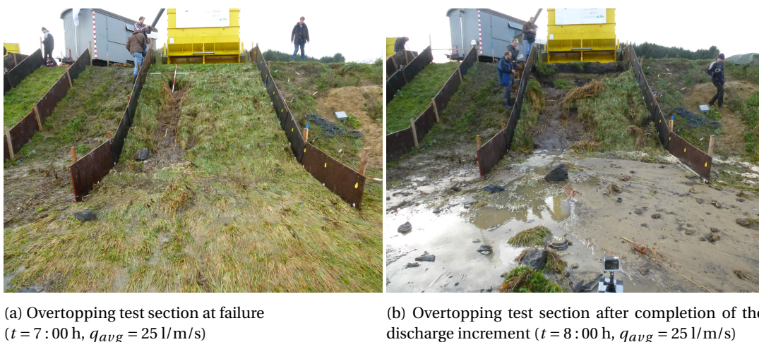
Figure 3.10: Damage observed after incrementally increasing overtopping tests at the Wijmeerspolder
