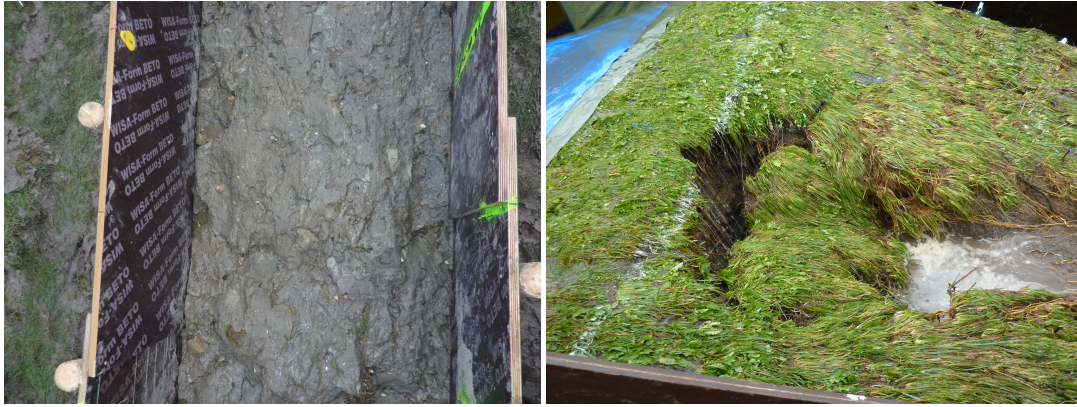
(a) Surface erosion observed during overflow tests on sand (after: Yagisawa (2019a), see Chapter 3)
