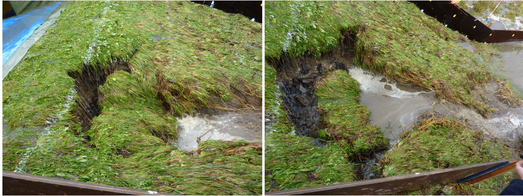
(a) A steep headcut during overtopping (top view)
