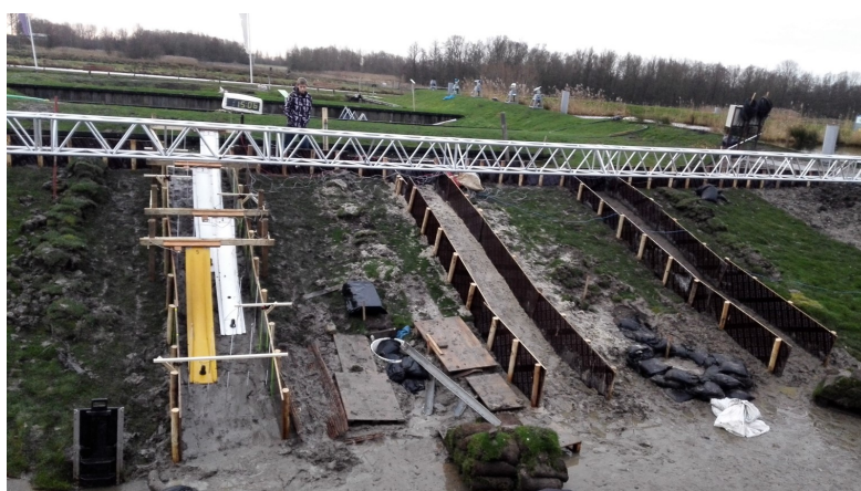
Figure 3.3: Viewpoint Flood Proof Holland overflow test sections
