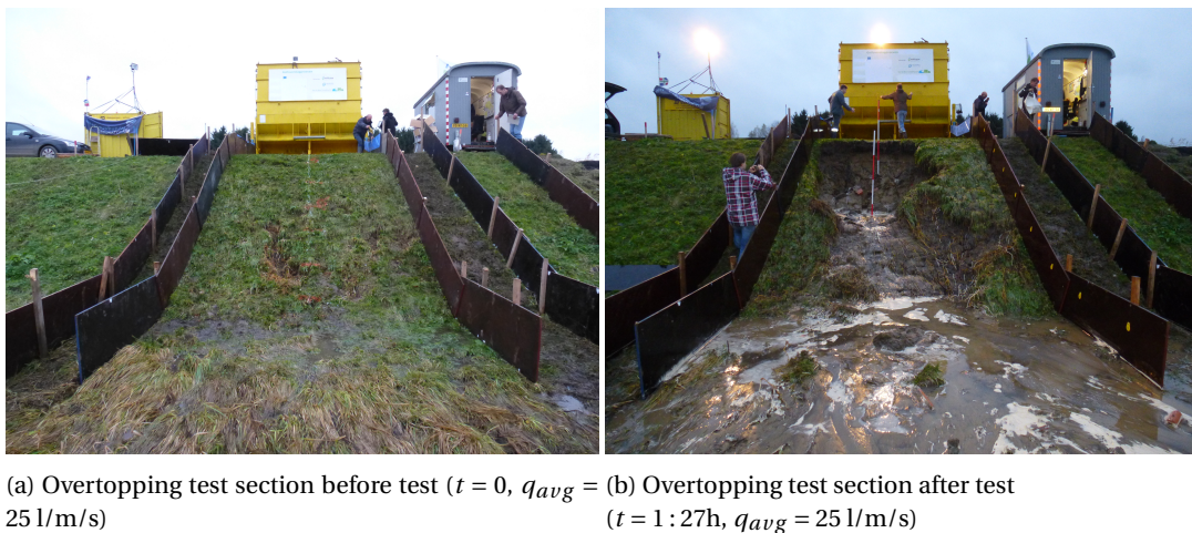
Figure 3.8: Damage observed after continuous overtopping tests at the Wijmeerspolder
