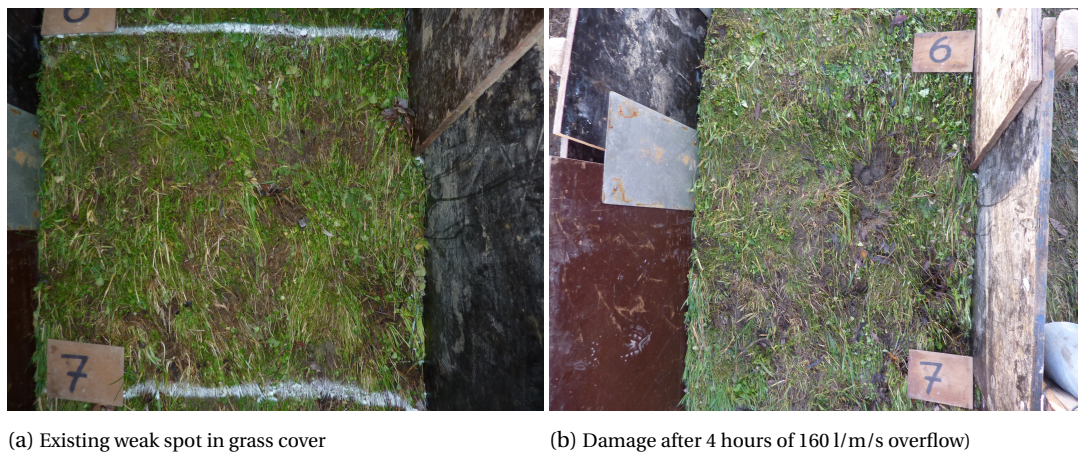
Figure 1.5: Failure of a grass cover near a weak spot during overflow (after: Bakker and Mom (2015b), see Chapter 3)
