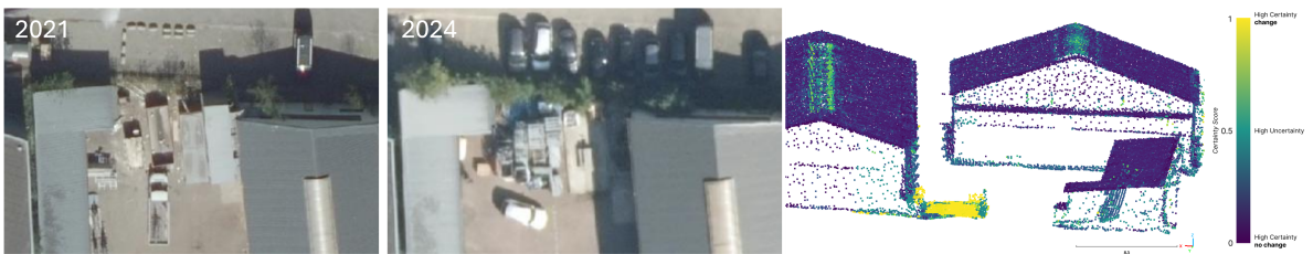
Figure D.7.: Removal of a building section detected between AHN4 and AHN5. The ground points in the former building footprint show high change probability, accurately reflecting the structural disappearance. Orthophotos from 2021 and 2024 are provided for context, source: Beeldmateriaal Nederland .
