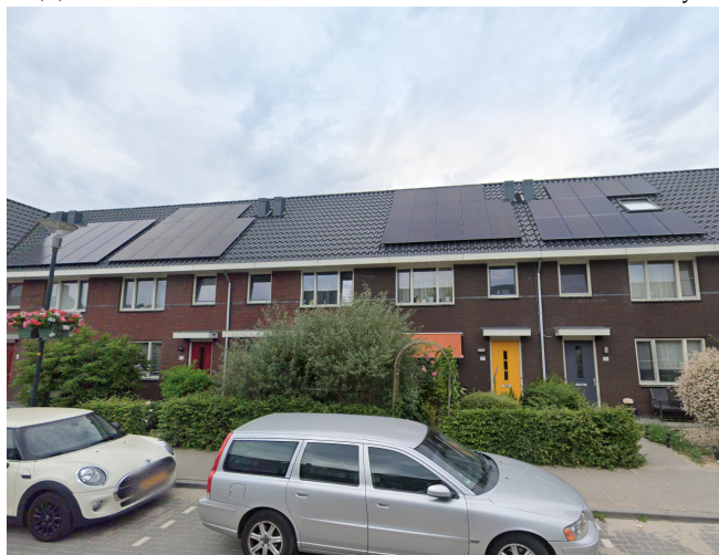
(c) Street view from Zaltbommel showing solar panels. Source: Google [2021].
