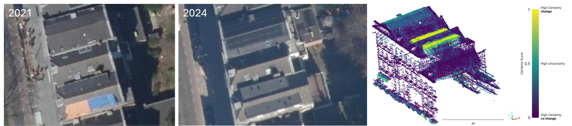
Figure D.18.: Change detection result showing a dormer added between AHN4 (reference point cloud dataset) and Rotterdam 2024 (target point cloud dataset). The added structure is clearly detected with high certainty of change. Orthophotos from 2021 and 2024 are included for context. Source: Beeldmateriaal Nederland .
