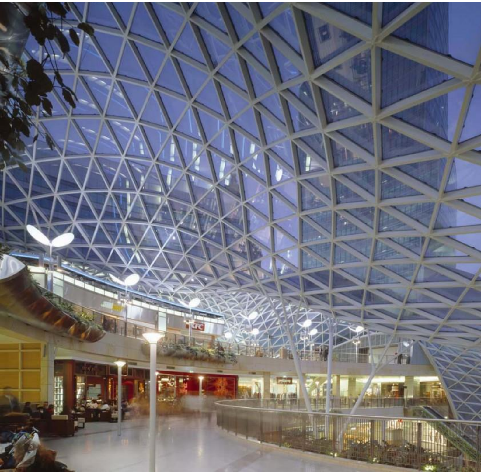
Figure 4-14 Interior view of Zlote Tarasy atrium roof (Anderson & Czajewski, 2008)
