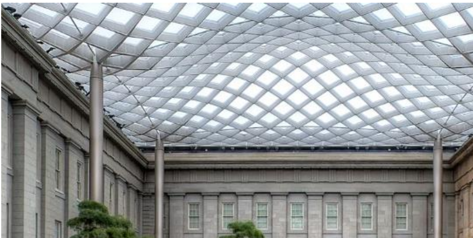
Figure 4-17 Example project with warped planar quad glass panes on the inner courtyard of the Portrait Gallery roof, Washington DC (Foster and partners)
