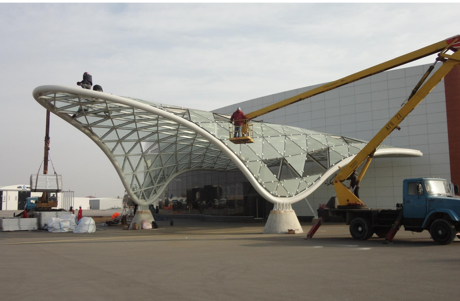
Figure 6-1 The freeform canopy at Baku international airport in construction process
