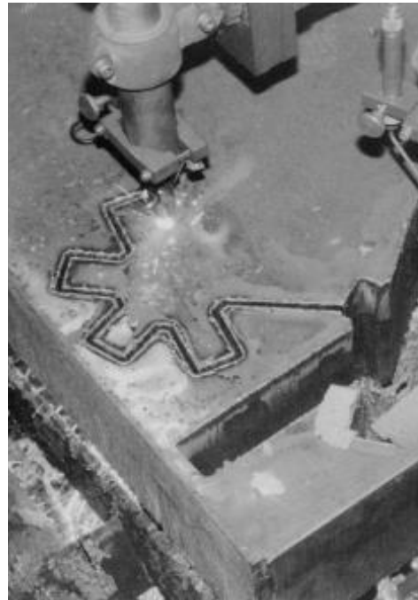
Figure 4-8 Cutting of nodes out of steel plate 180 mm with CNC machine
