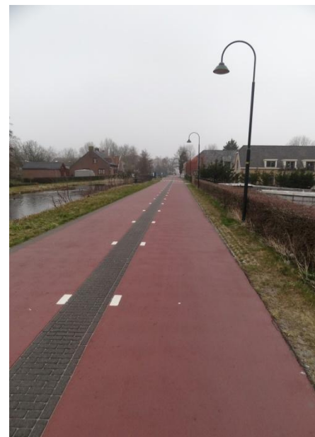
FIGURE 45: URBAN PROFILE OF THE TWO-LANE BICYCLE STREET IN ZOETERMEER. THE BICYCLE STREET LIES WITHIN THE BUILT-UP AREA.
