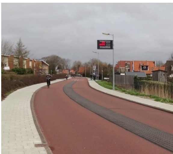
FIGURE 21: A TWO-LANE BICYCLE STREET WITH A WIDE PROFILE WHERE CYCLISTS CHOOSE TO DRIVE ON THE RIGHT-HAND SIDE OF THE ROAD.
