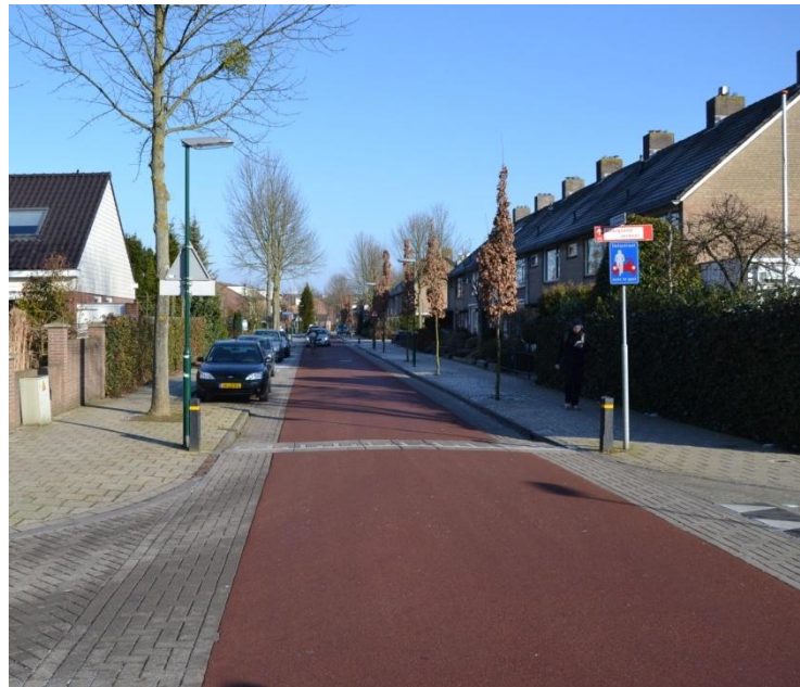
FIGURE 53: THE SINGLE-LANE BICYCLE STREET AT THE PRINSES IRENEWEG IN HOUTEN
