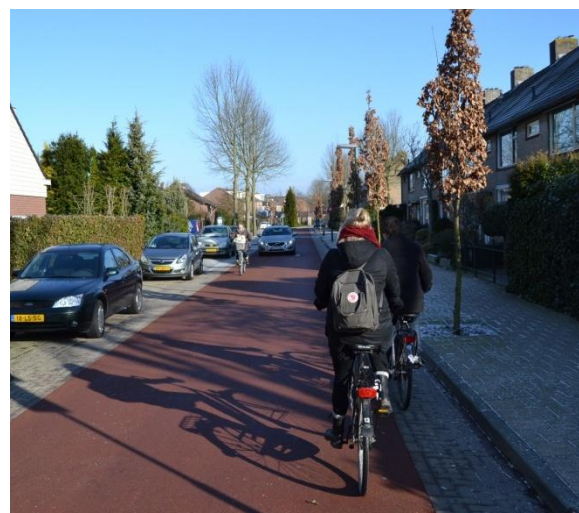
FIGURE 22: A NARROW SINGLE-LANE BICYCLE STREET, WHERE THE CAR HAS TO STAY BEHIND THE CYCLIST SINCE THERE IS NO SPACE TO PASS THE CYCLISTS.
