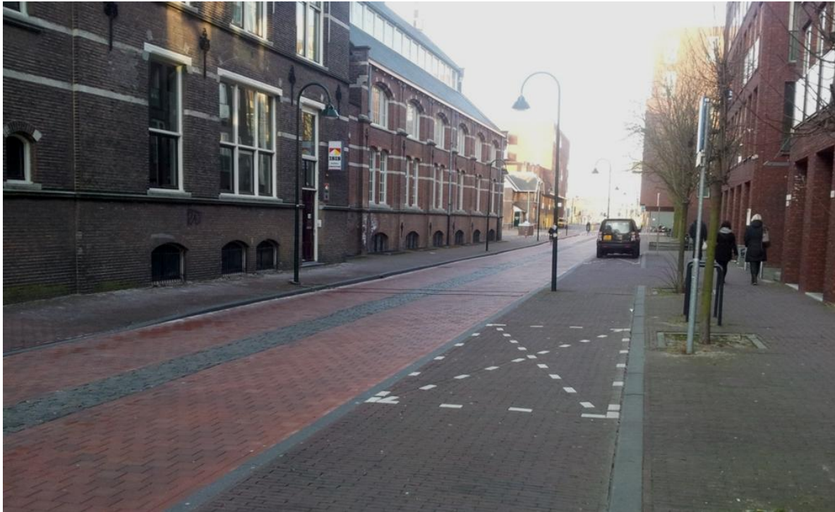
FIGURE 42: TWO-LANE BICYCLE STREET AT THE EZELSVELDLAAN IN DELFT, HAVING OLD BUILDINGS ON ONE SIDE AND NEW BUILDINGS ON THE OTHER SIDE. THE PARKING DEMAND IS FACILITATED BY PARKING SPOTS ALONG THE BICYCLE STREET.
