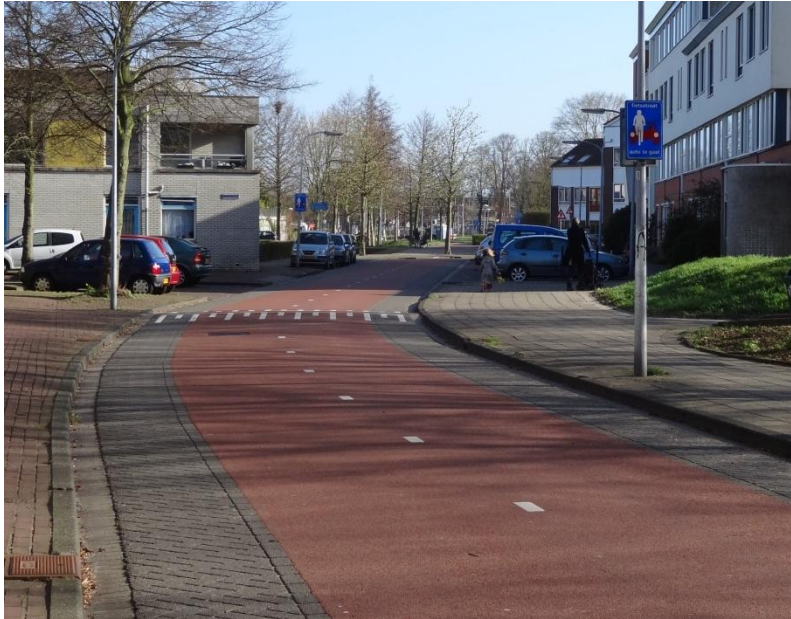
FIGURE 18: BICYCLE STREET IN HAARLEM WITH BICYCLE PATH LANE LINE IN THE MIDDLE OF THE STREET. THIS LANE LINE HAS BEEN ADDED LATER, WHEN AN EVALUATION AMONG USERS SHOWED THAT THE DESIGN WAS NOT CLEAR ENOUGH. THE APPLICATION OF A LANE LINE STRENGTHENED THE ASSOCIATION WITH A BICYCLE PATH.
