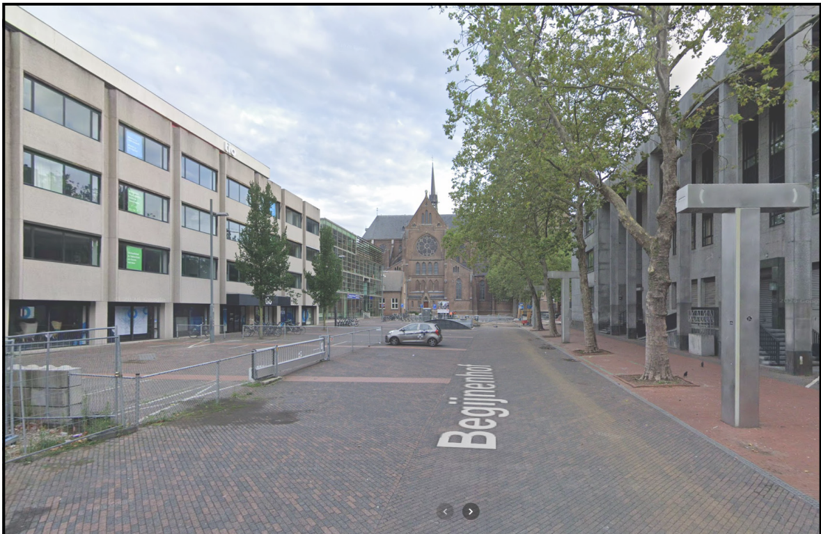
Google Street View image of Begijnhof, showing its current condition.
