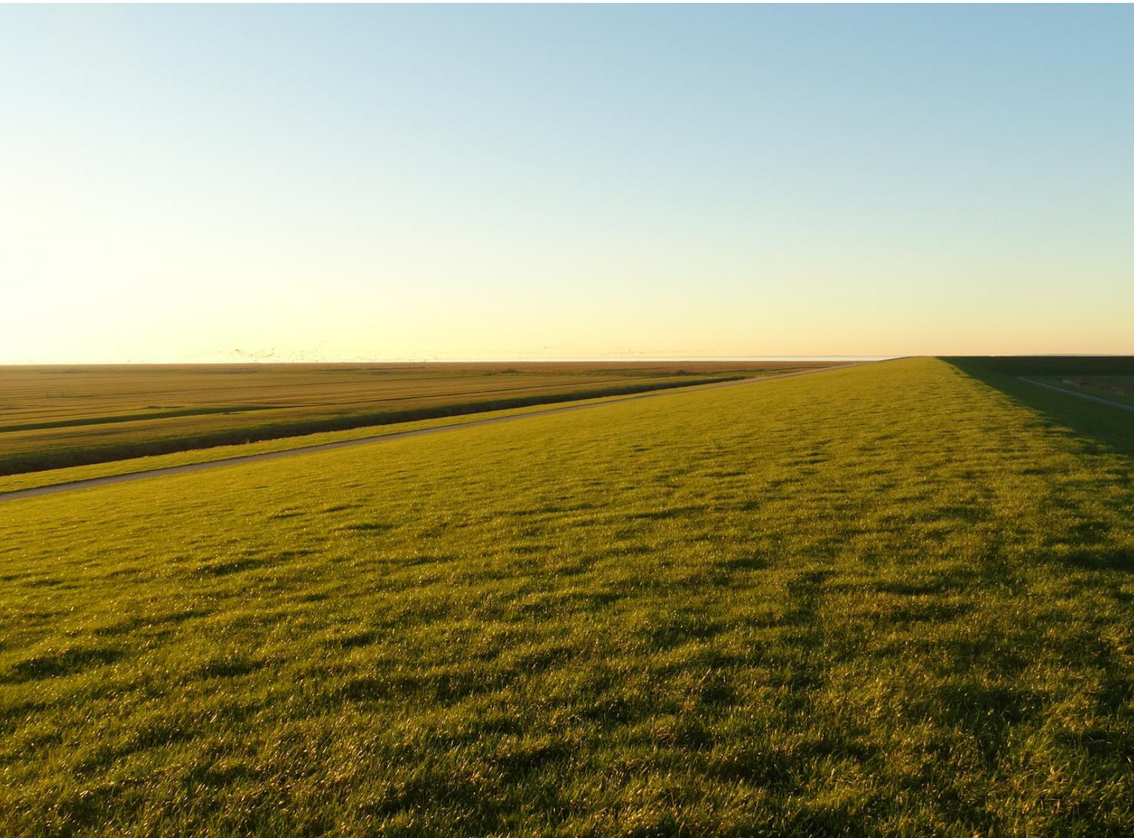
Sea dike Friesland
