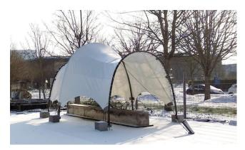
Figure 2.6: F.A.B. Shell by ENPC, 2020: Assembled formwork prototype [37]
