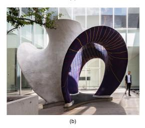
Figure 2.7: KnitCandela shell by Block Research Group and the Computational Design Group of Zaha Hadid Architects, 2018: (a) Construction and (b) finished shell structure (Photo credits: (a): Mariana Popescu, (b): Angelica Ibarra)
